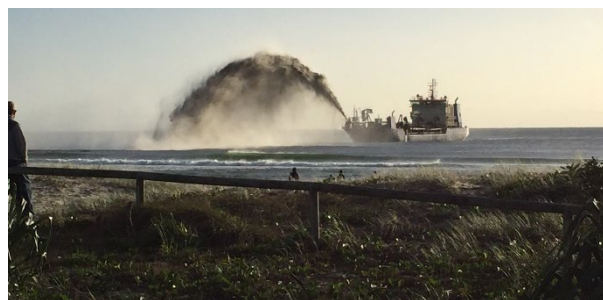
Figure 3: Rhode Nielsen Balder R rainbowing during the 2017 Gold Coast Beach Nourishment Project.
